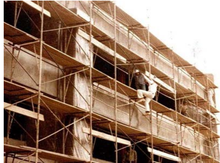
Do not access by cross braces
