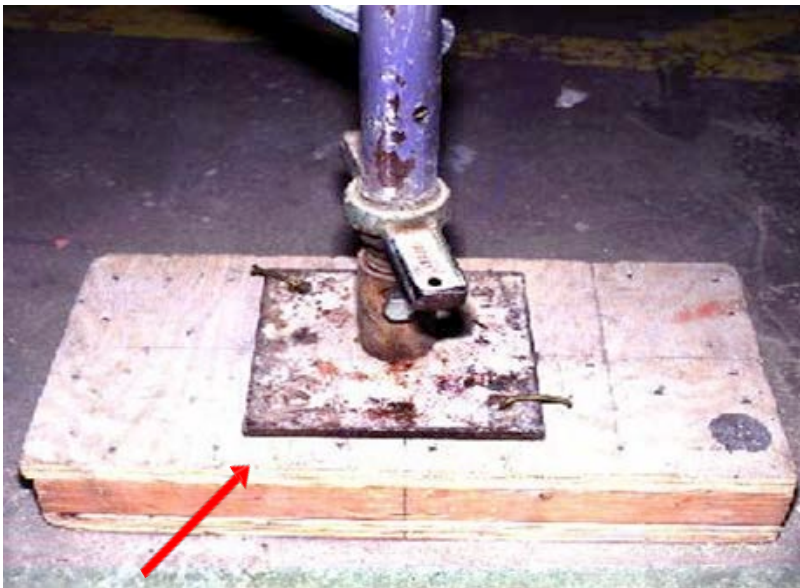
Base Plate An example of good support
